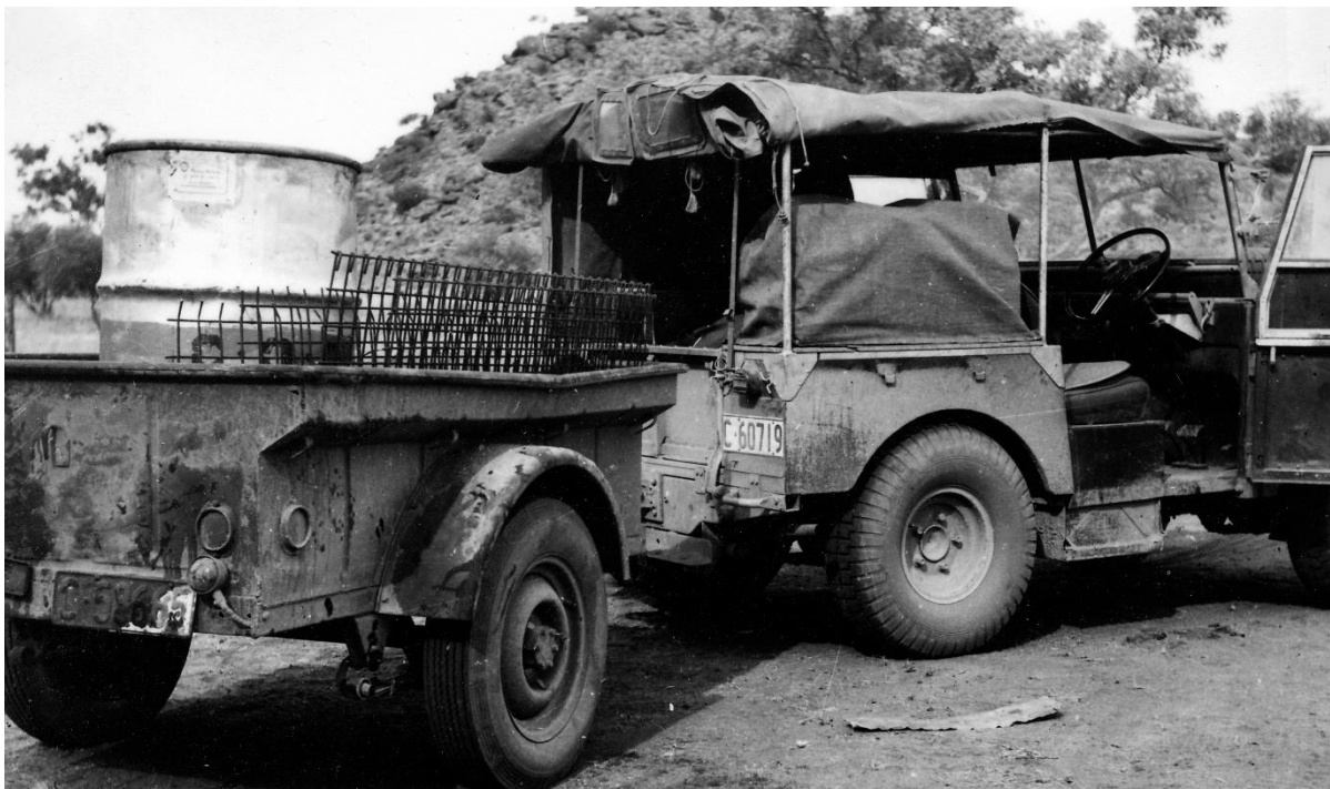
Figure 9. Short-wheel base Land Rover and Jeep trailer. Note the 900 x 13 tyres on the Rover and the wireless dust cover.
