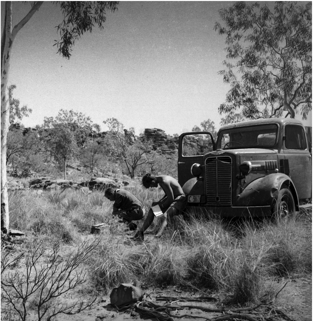
Figure 5. Reading the Aneroid Barometers. Note headlamps on the Commer truck turned aside to protect the glass and bulbs. (Dave Hocking reading and Eric Crisp booking, at site between Robinson River Homestead and Calvert Hills Homestead, 1949 – Ed.)
