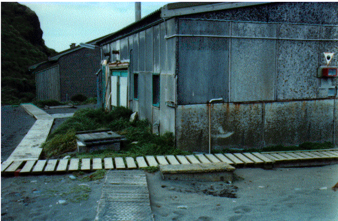
Service Pits - near Emergency Power House
