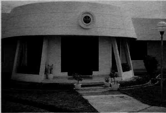
LAPAN headquarters at Pare Pare.
